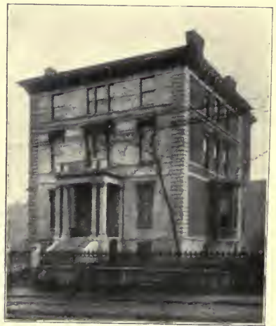
THE BRANT RESIDENCE On Chouteau avenue. Headquarters in war times, now a factory
